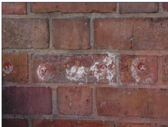
Figure (4) Shows horizontal insulation incorrectly made with water glass and cement (photo by the author)
