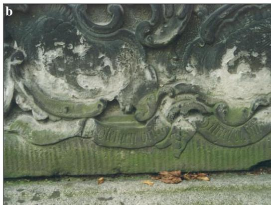
Figure (6) Shows **a.** architectural detail from Gotland sandstone, disintegration of stone under corrosive layers (photo by the author), **b.** fragment of the epitaph of Gottfried Mentzl and his wife Anna Rosina, disintegration of stone (sandstone with silica-loam sand binder) under the layers, action of salt and microorganisms (photo by W. Domasłowski)
