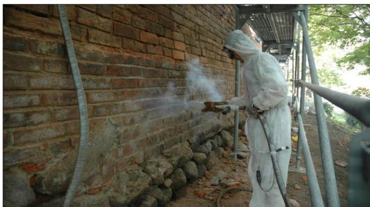
Figure (11) Shows dry ice cleaning, freezing of a damp wall (photo by the author)
