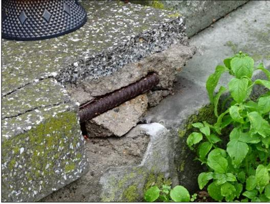
Figure (7) Shows architectural detail destroyed as a result of material stress caused by corrosion of steel elements (photo by the author)
