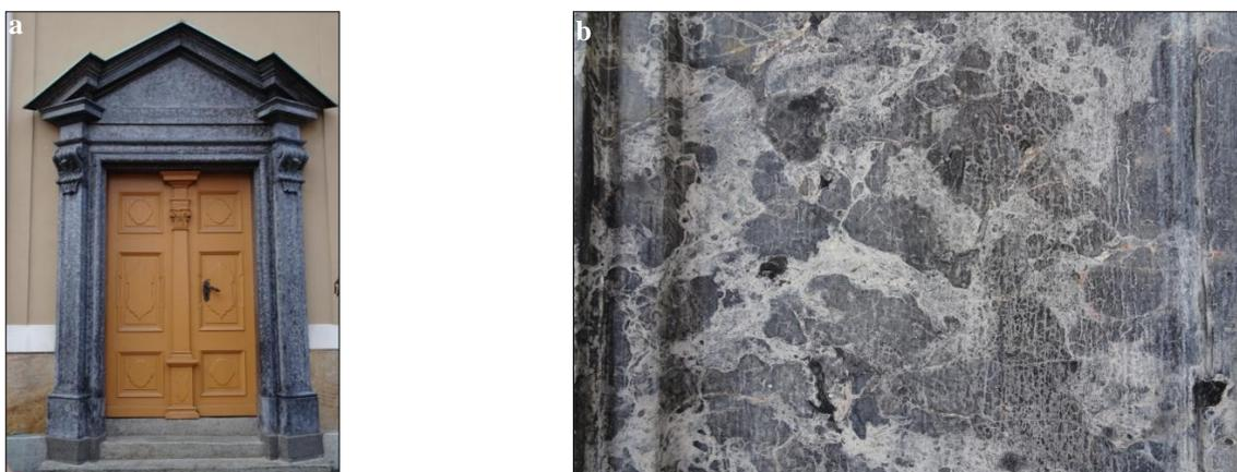
Figure (2) Shows **a**. Toruń, church of the holy spirit, southern elevation, portal made of compacted limestone from Dębnik, **b**. Dębnik fragment (photos by the author)
